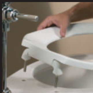
Assemble hinges.
